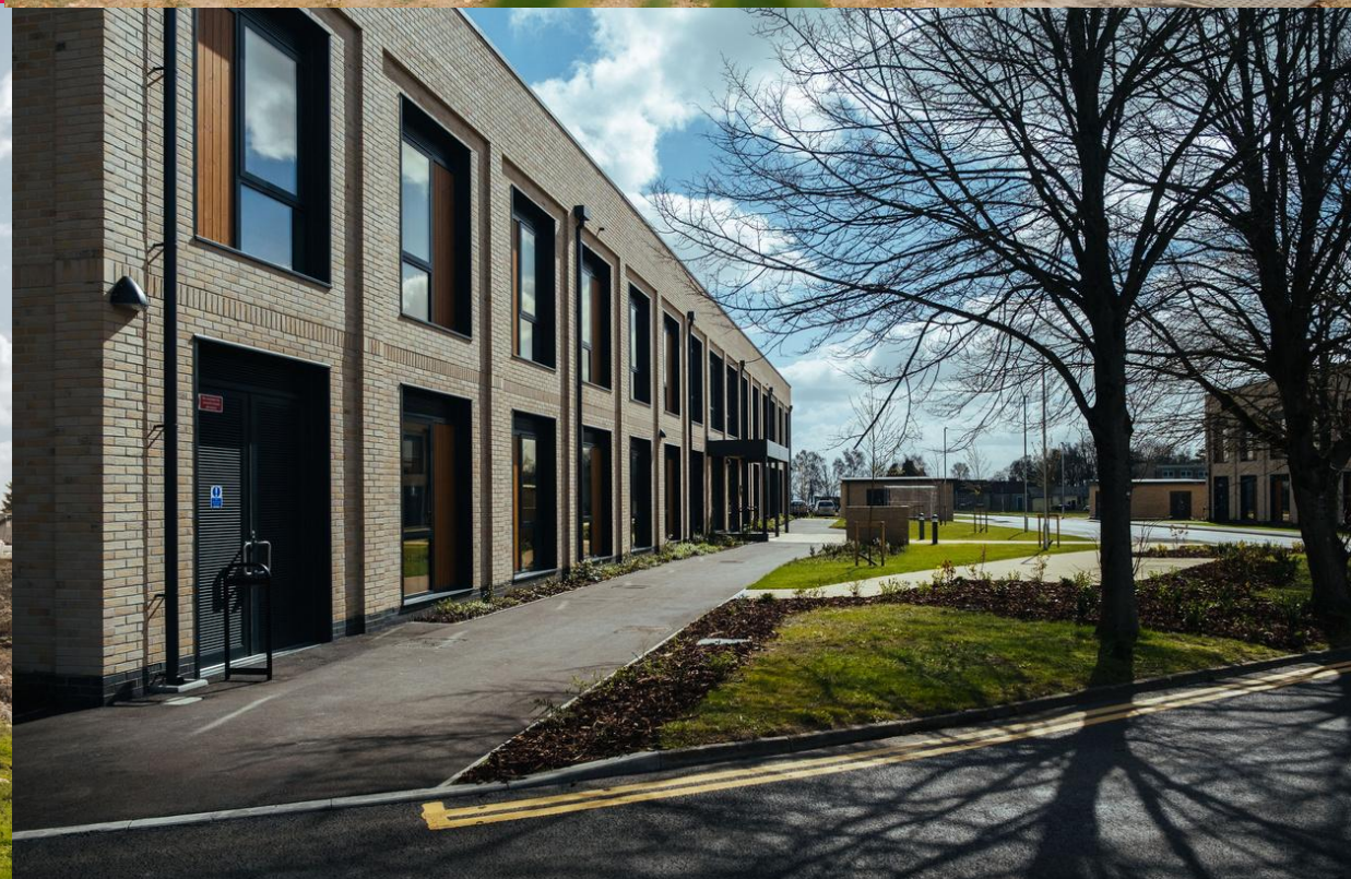
11 SCHEMES IN PRE-CONSTRUCTION
