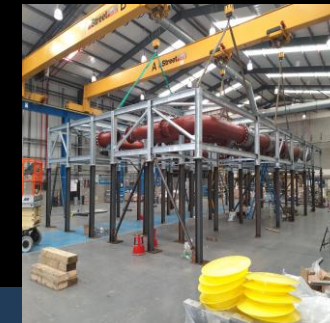
Interstitial Plant Decks
