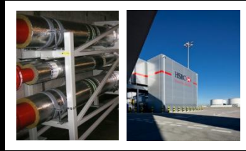
Heathrow Terminal 5C Tunnel and Nodes
