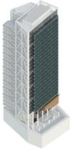
South and West Brise Soleil
