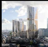
2 Finsbury Avenue British Land
